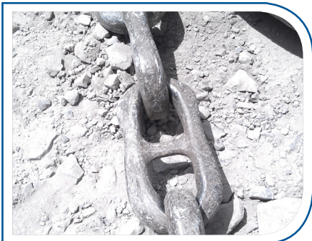
3" Hoist Chain prior to being removed
